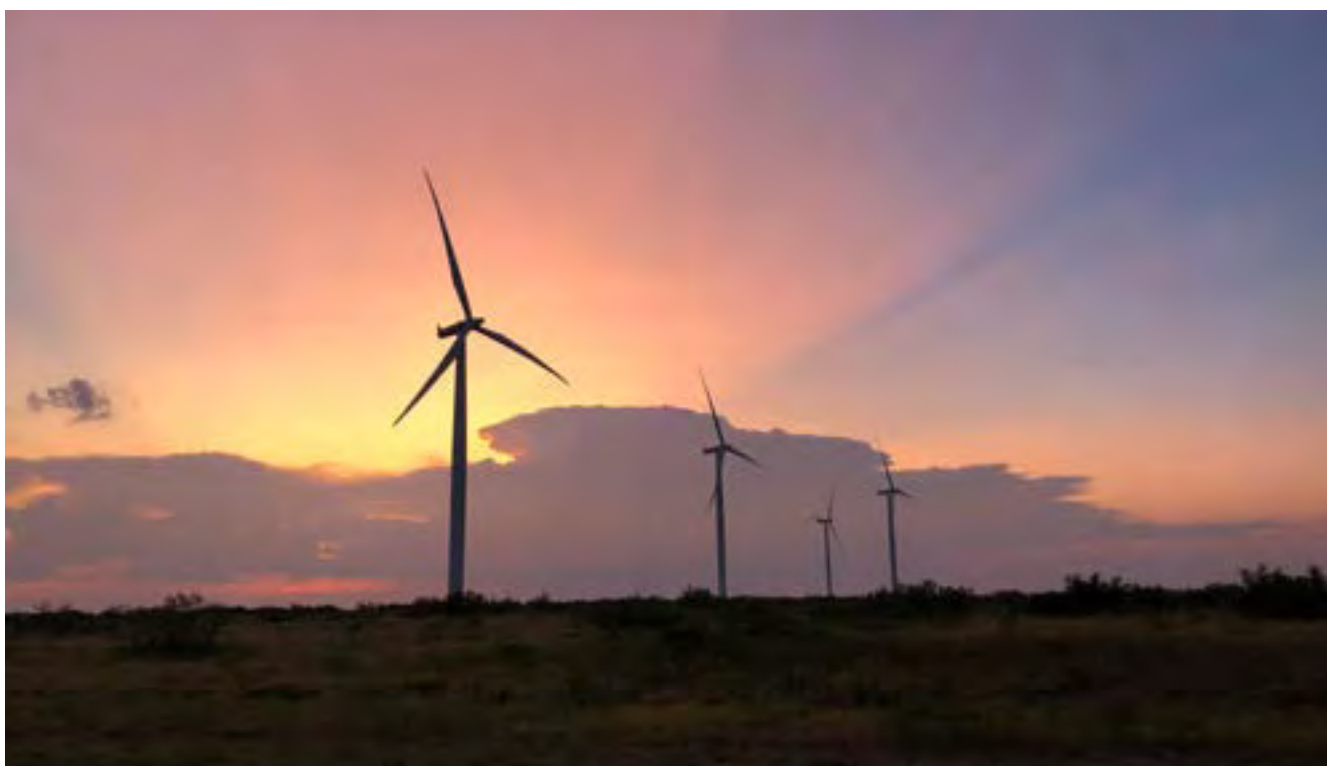
Whirlwind 60 MW wind project in Texas
