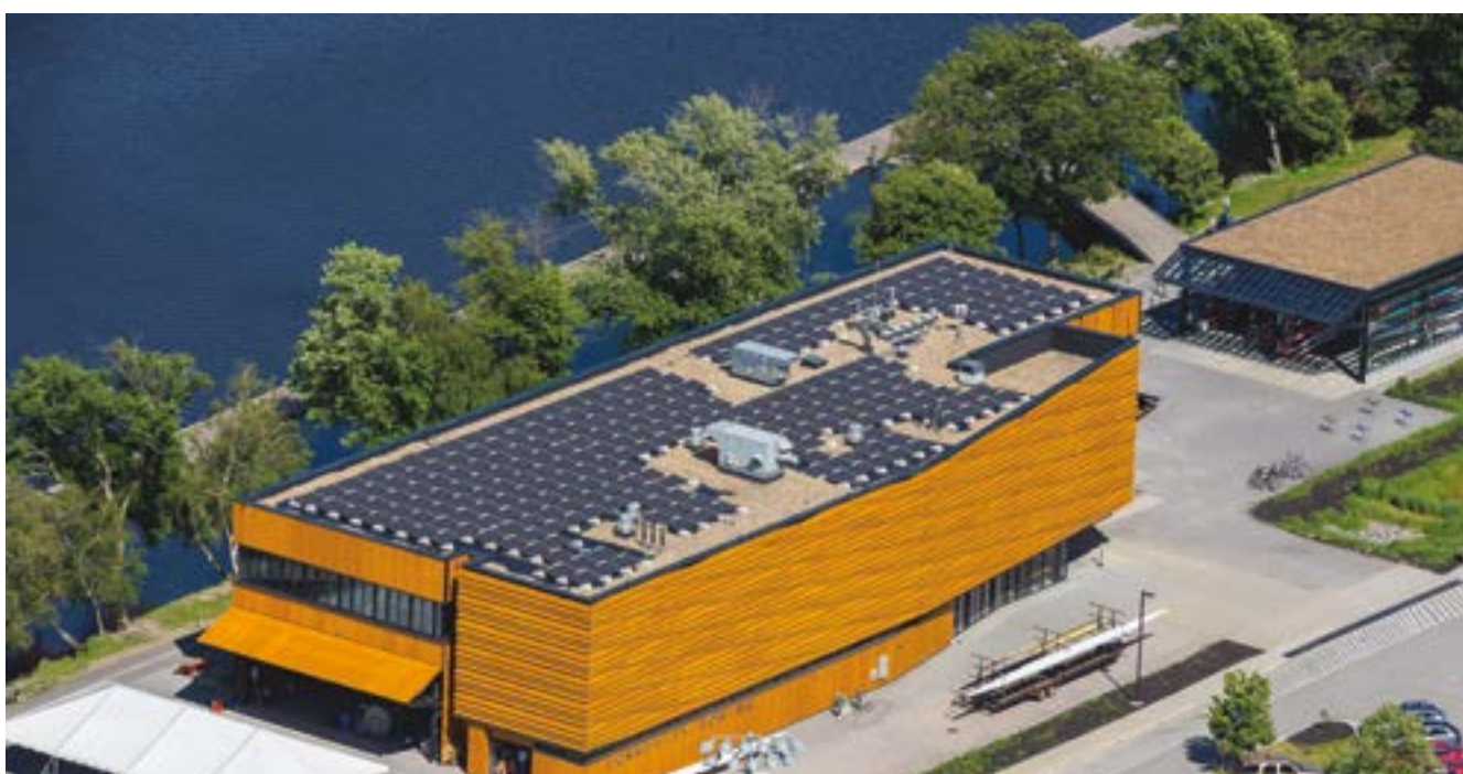
Rooftop solar system at a community rowing facility in Massachusetts, part of SED Solar Portfolio
