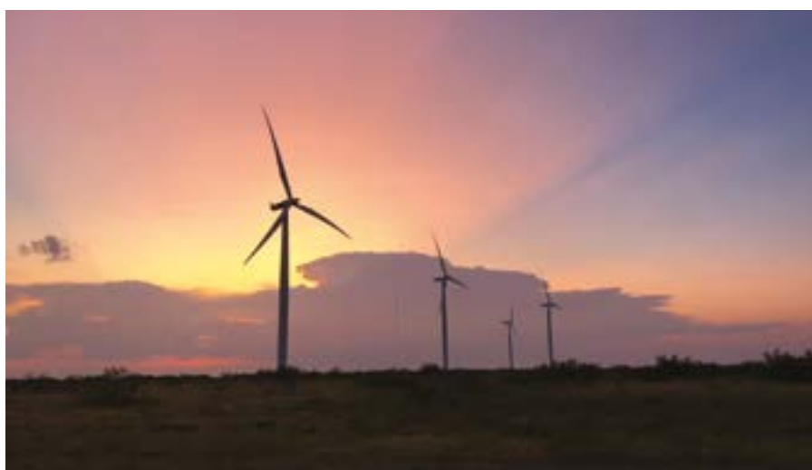
Whirlwind 60 MW wind project in Texas
